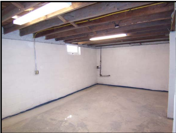
Ready To Finish Basement
